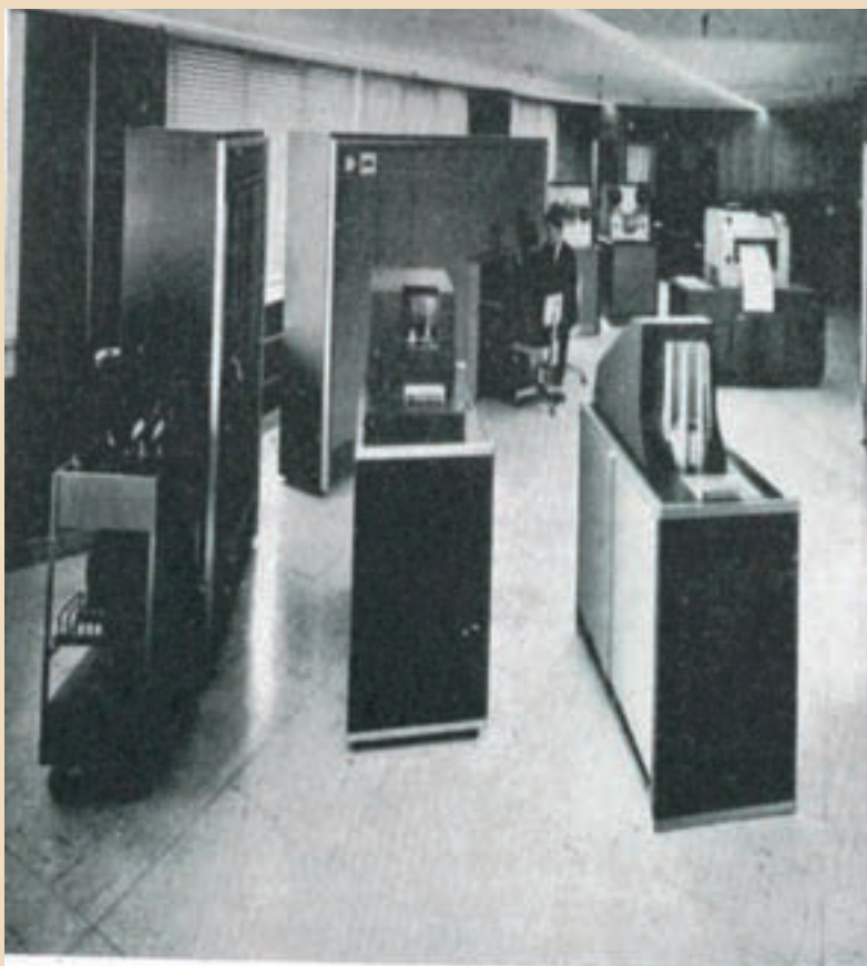
A typical I.C.T. 1300 Computer installation. On the left is the Magnetic Tape Unit with the Control Processor (and Console), Paper Tape Reader and Punch, and High Speed Printer in the background. The Card Punch and Card Reader are shown in the foreground. This I.C.T. 1300 EDP System forms part of the company's new data processing system in North Australia.
